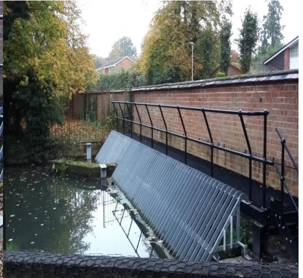
Figure 12: New trash screen during normal conditions
