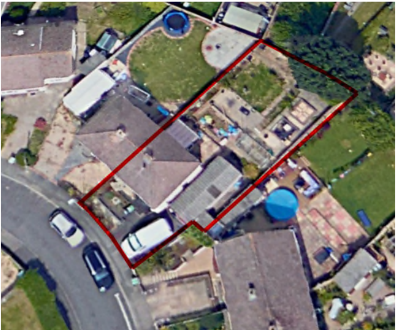
View of site looking over the property
