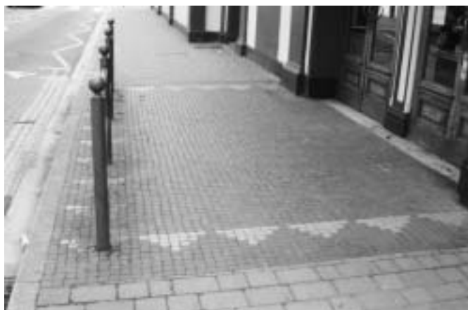
Pattern in footway outside New Olympus Theatre.
