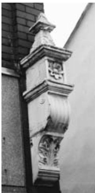
Example of corbel attached to no. 155 Barton Street.
