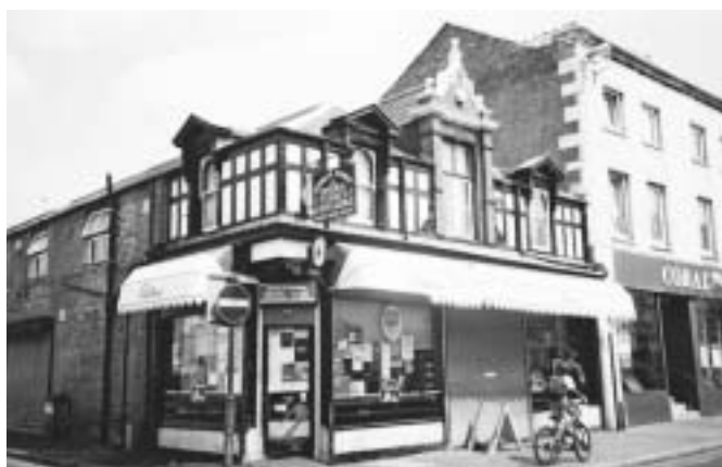
Douglas Stores, 125 to 129 Barton Street.
