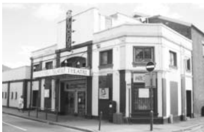
New Olympus Theatre (grade II).
