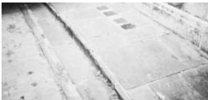
Stone paving beside Gothic Cottages.
