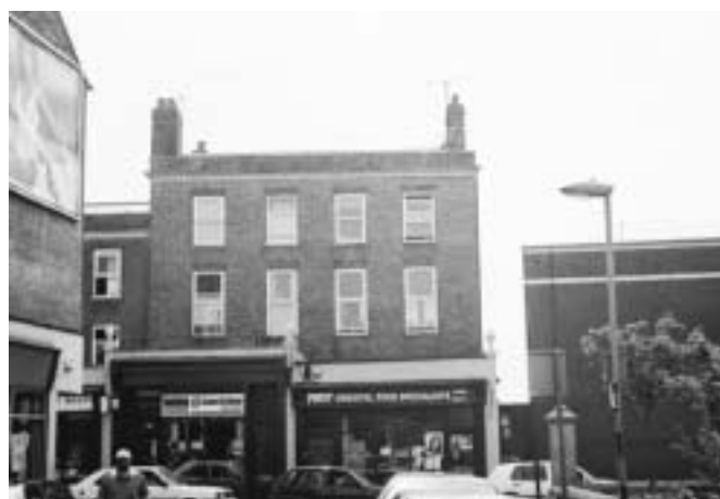
Nos 110-112 Barton Street (grade II).
