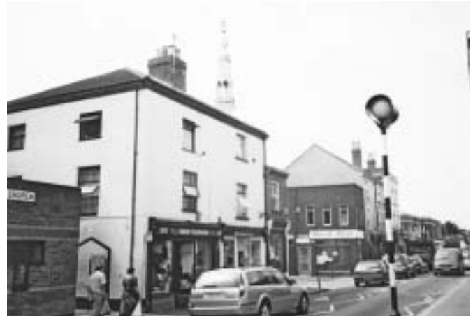
Looking east along Barton Street (south side).
