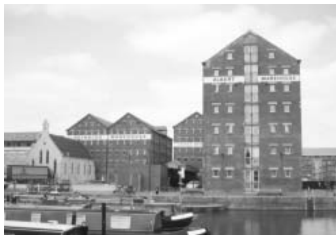
Albert Warehouse towering above The Mariners' Church.
