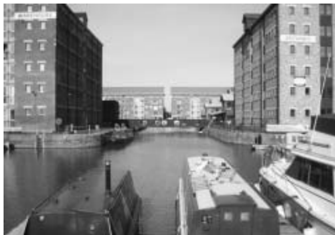
New development framed between Albert and Britannia Warehouses.
