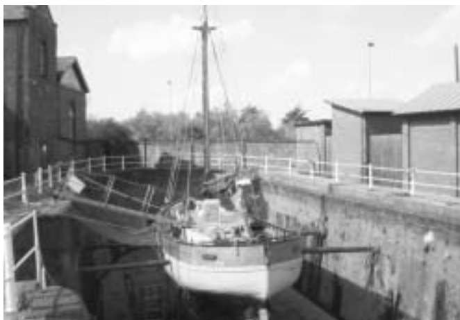
The smaller of two 19th century dry docks west of the main basin.
