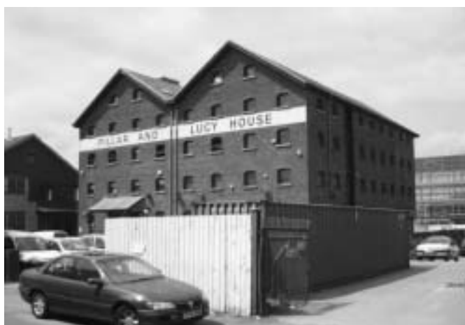
Merchants Road frontage of the Pillar and Lucy Warehouse.
