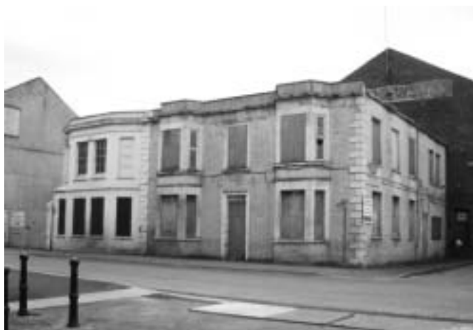
Sudbrooke House, Llanthony Road (south side).
