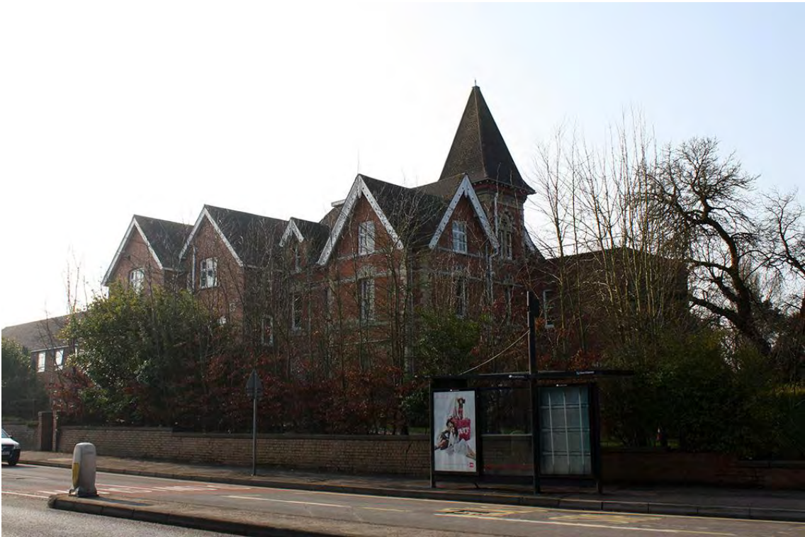
Plate 1: Bohanam House from the north east
