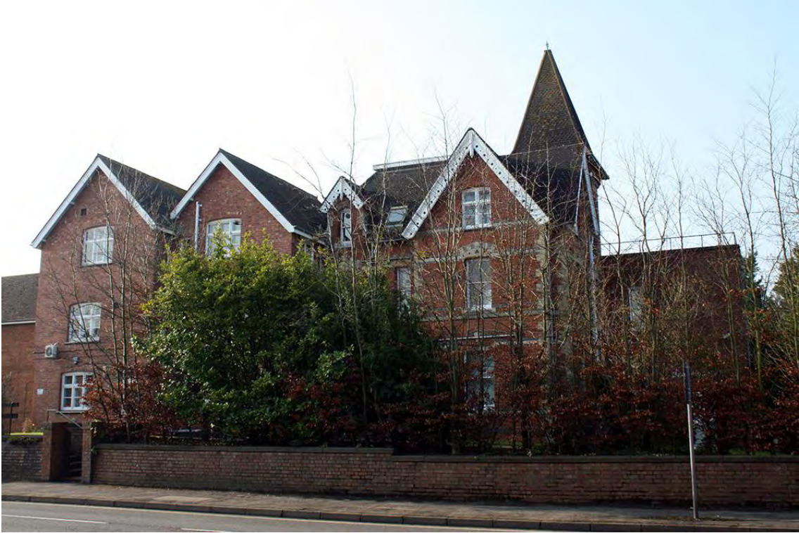
Plate 2: Bohanam House from the north
