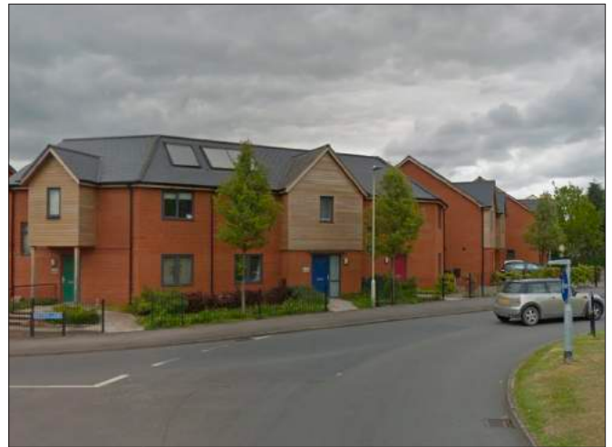
Fig 5.2: New houses: There is no 'left over' space: the front gardens have a clear role in providing separation from the street. The buildings are designed to 'turn the corner', with windows and bays looking outwards over the street. The strong building line helps define the street.
