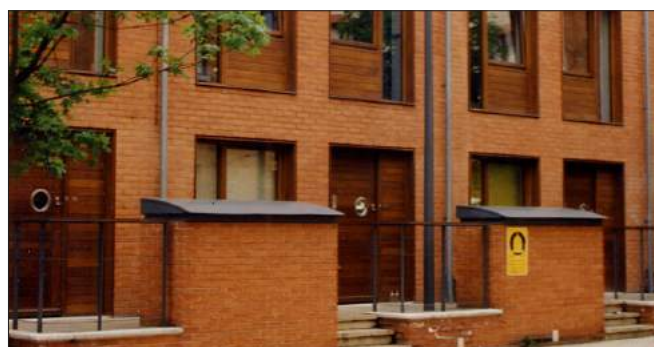
Fig 5.28: Bin storage positively designed into boundary treatment.
