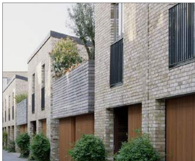
Fig 5.24: Windows and doors set back from the external facade give a building ‘depth’, avoiding a flat appearance.
