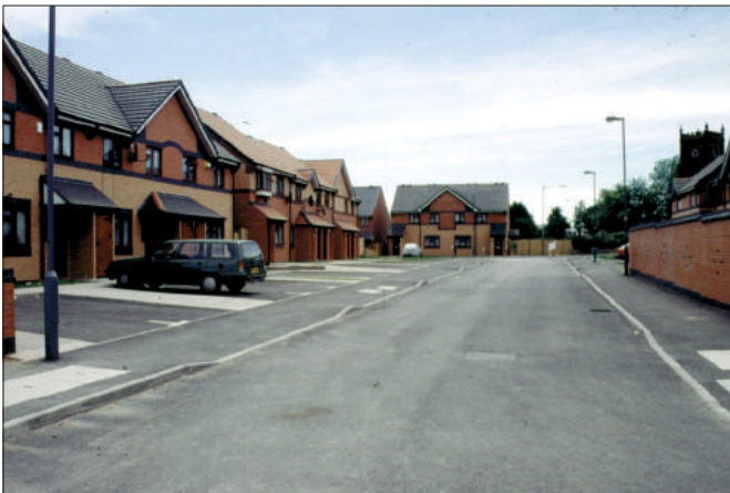
Fig 5.11: What not to do: parked cars and tarmac dominating the street scene.
