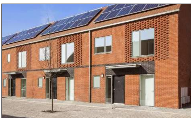
Fig 5.26: Textured brickwork provides robust three-dimensional interest that will stand the test of time
