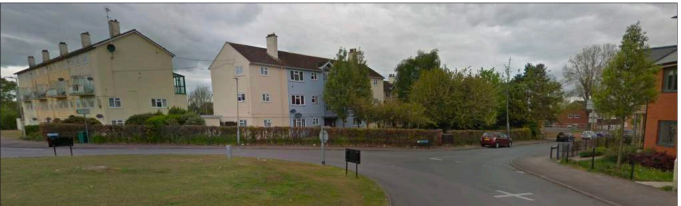
Fig 5.3: Older flats: Arranging the flats at right angles to one another on a curving corner results in 'left over' space, with no clear function, between the flats and the street. The blank gable end doesn't look good in such a prominent corner location.
