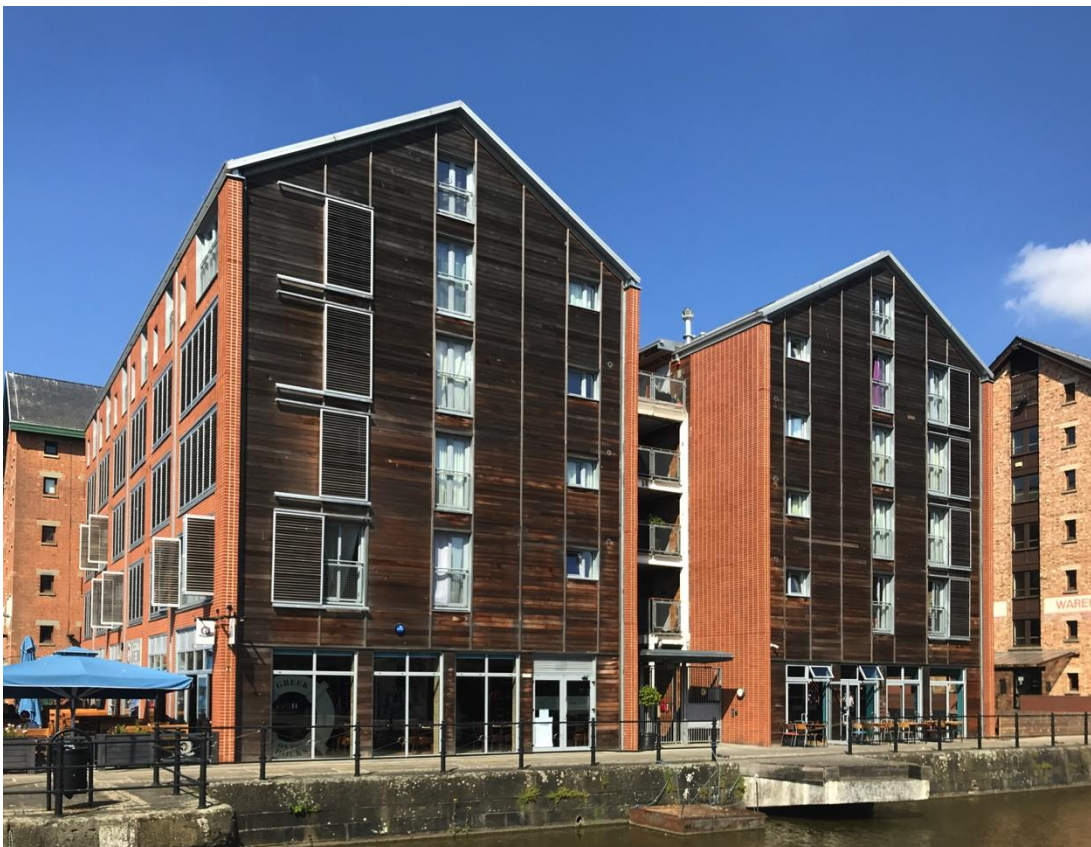
Merchants Quay – Residential development with commercial units below.
