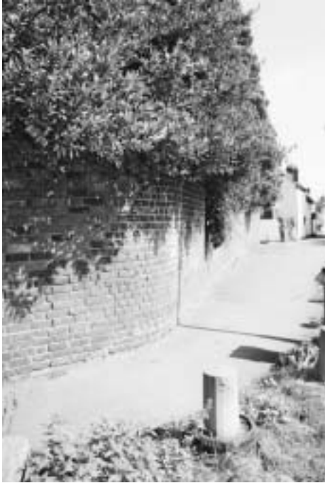
Positive: historic red brick boundary walls.
