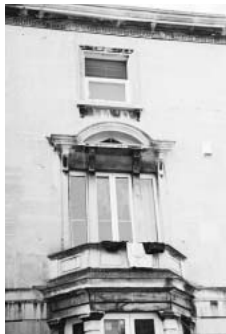
Nos 13 and 15 Kingsholm Road have particularly ornate street elevations, with Greek key design in the eaves cornices and moulded stone window surrounds.
