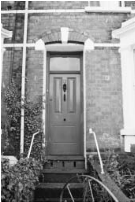
Stone steps and timber front doors, rectangular over door lights in Connaught Parade.
