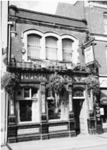
The tiled front elevation of the listed Imperial (No 59 Northgate Street) is a fine example of late-19th century pub design.
