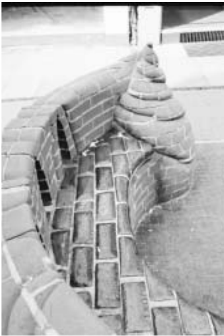
Rubbed brick and blue-glazed seating in memory of the Rt Revd Mgr Canon M J Roche 1899–1993.
