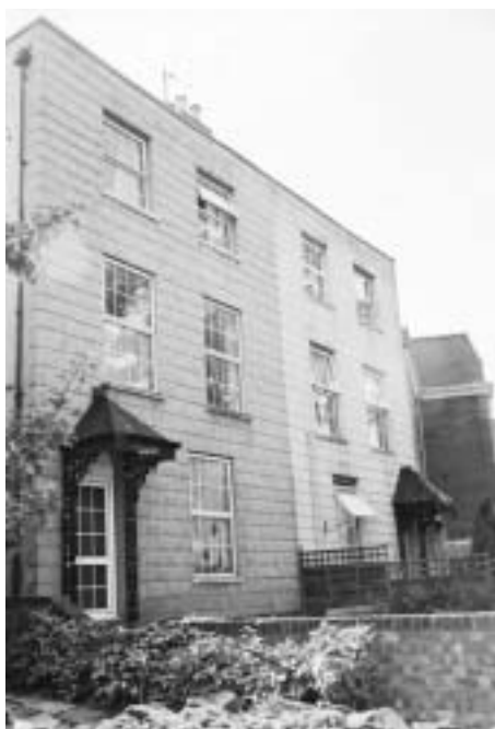
Erosion of historic character through the replacement of original timber sash windows or doors with uPVC alternatives.
