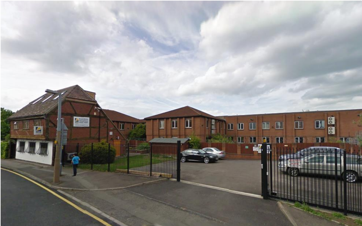
Plate 2: The SUB58 site from the south
