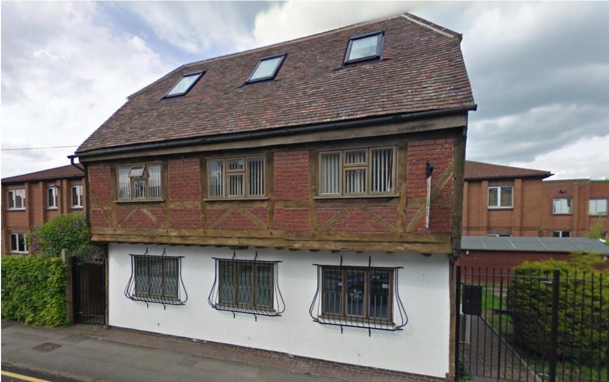
Plate 3: 30 St Catherine Street from the south
