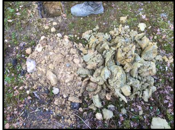
Starter pit arisings
