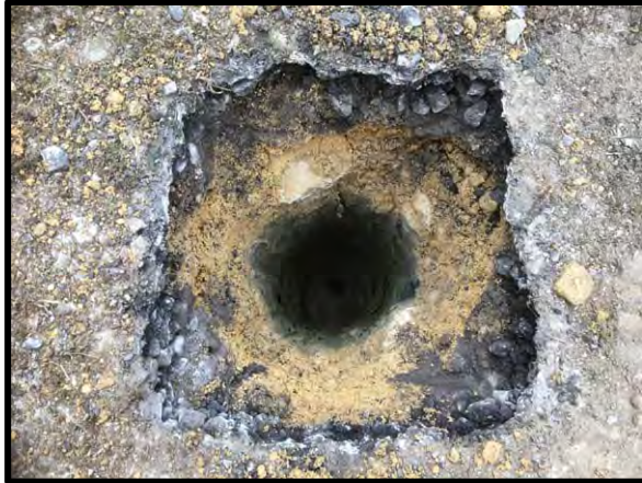
Hand-dug starter pit
