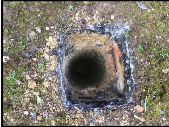
Hand-dug starter pit
