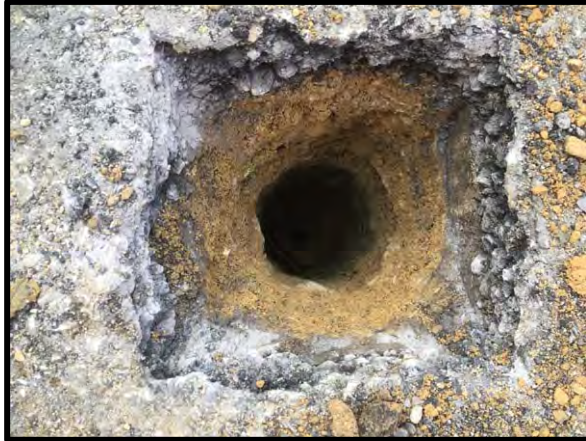
Hand-dug starter pit
