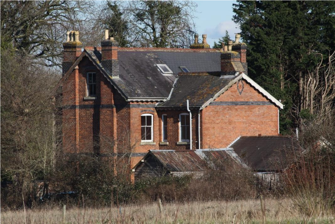
Plate 3: Fairfield Villa and Ferndale Villa from the south west
