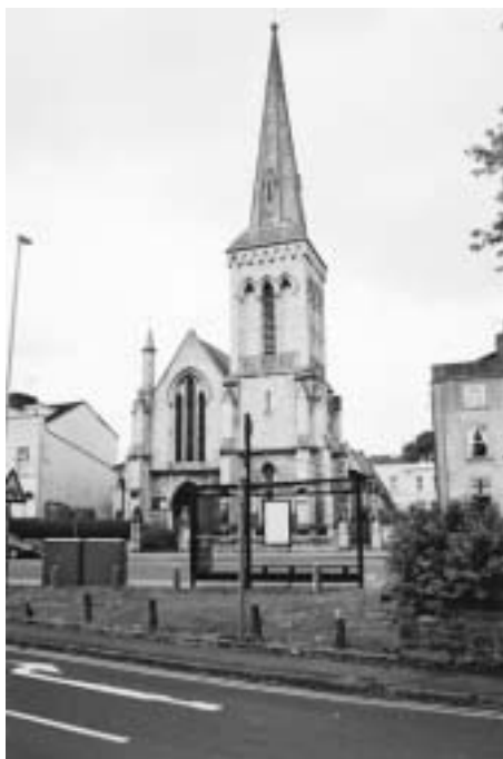
The spire of St Mark's Church is a prominent landmark.
