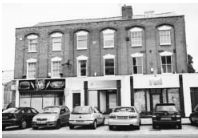
The characteristic Gloucester detail of flat-arched window heads of five raised-and-stepped stone voussoirs.
