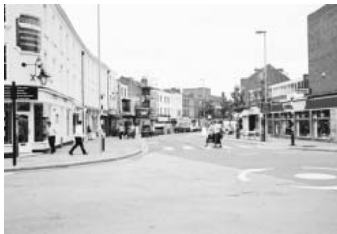
Worcester Street south of the railway viaduct.
