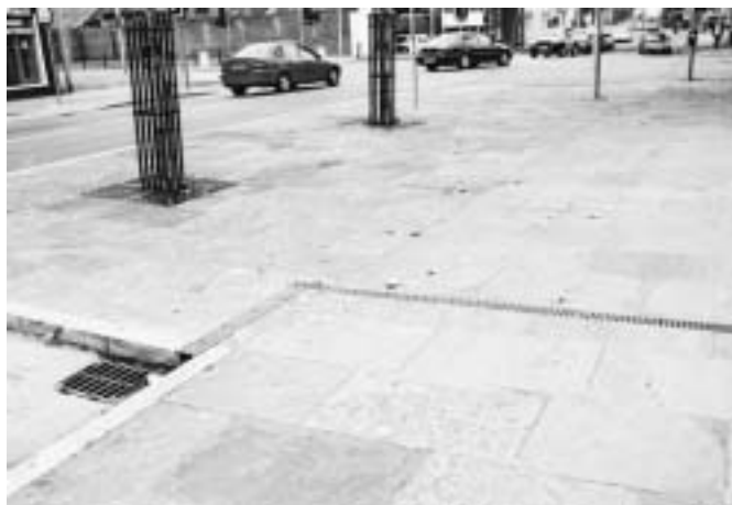
New paving and tree planting in the area covered by the Worcester Street Townscape Heritage Initiative.
