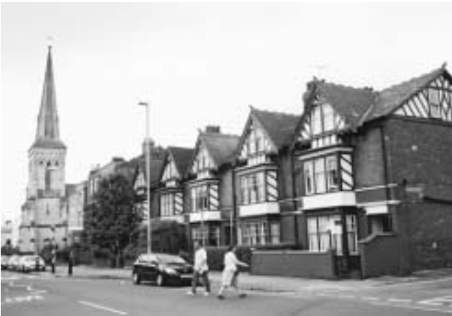
Nos 62 to 72 Worcester Street are attractive and flamboyant neo-Tudor dwellings designed by H A Lansley and built in 1904–7 that survive largely unaltered.
