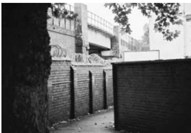
The unwelcoming appearance of the pedestrian alley leading to the County and Diocesan Records Office.
