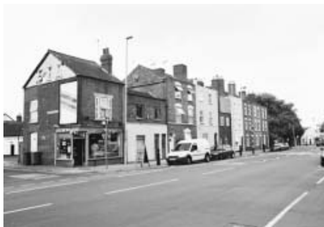
Worcester Street north of the railway viaduct.
