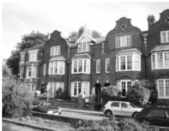
Nos 1 to 4 St Michael's Square.
