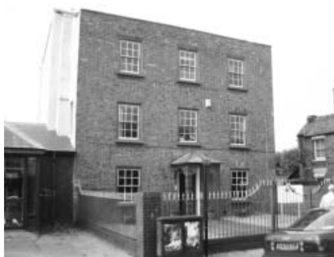
Ivy House, No. 94 Eastgate Street
