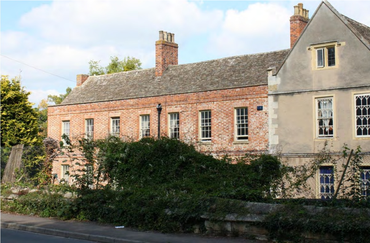
Plate 3: Matson House, adjacent to SUB41 site, from the west
