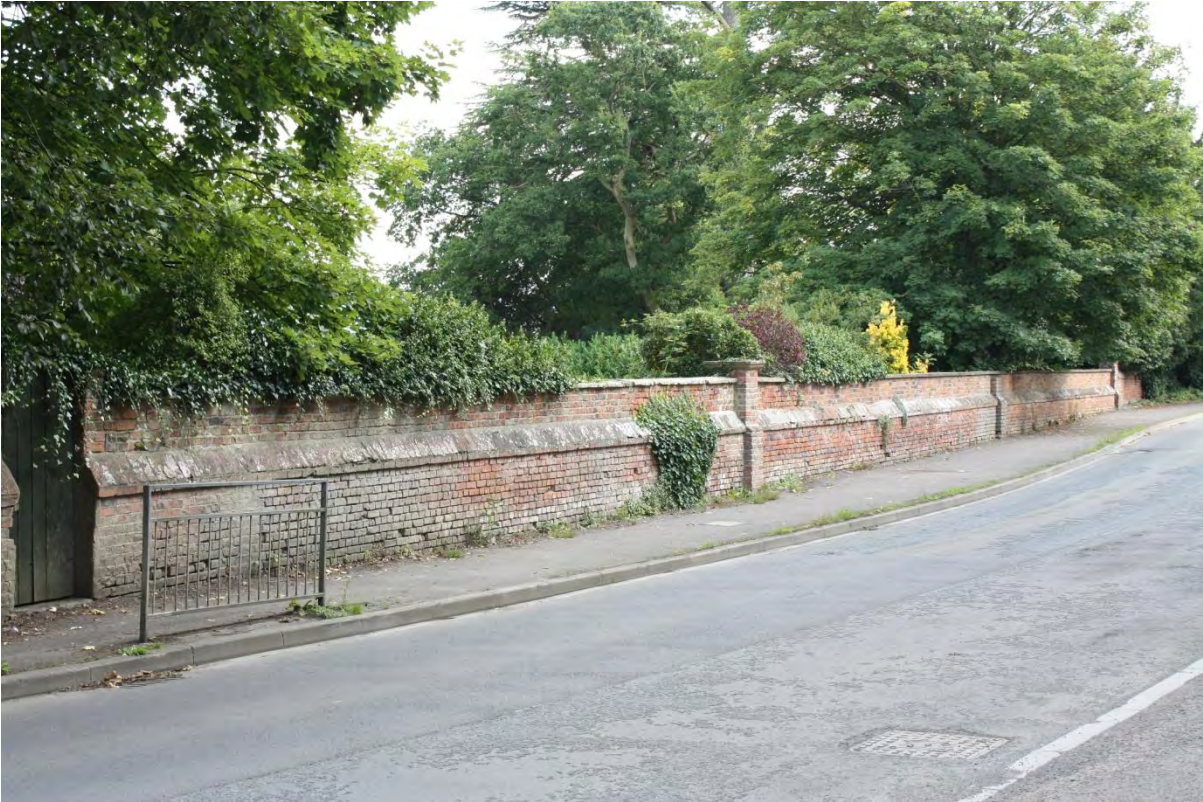
Plate 1: Garden wall on Matson Lane, boundary to SUB41 site
