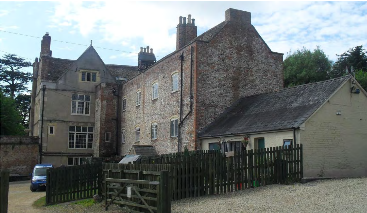
Plate 4: Matson House, adjacent to SUB41 site, from the east
