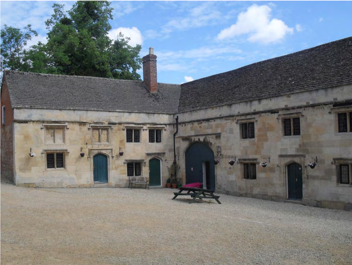
Plate 6: Former stables, adjacent to SUB41 site, from the east
