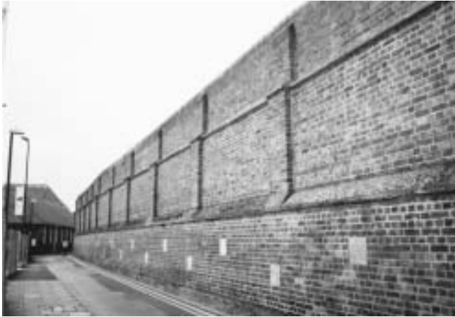
Parts of the wall around the prison, listed grade II.
