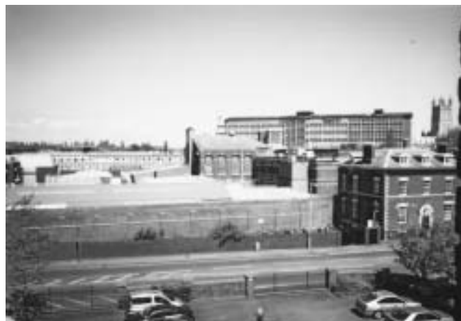
View over Gloucester Prison showing The Governor's House.
