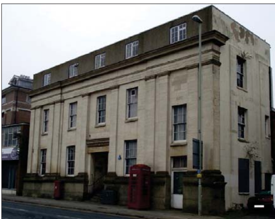
Albion House former C19th hotel with additional storey
