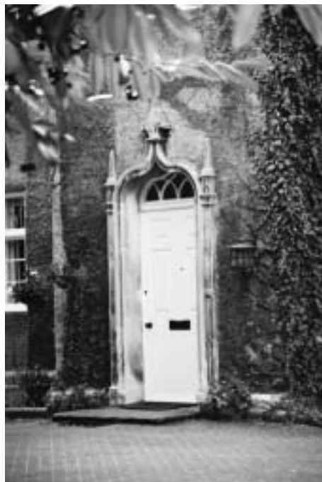
The 18th-century Gothick Coade Stone front door surround at Hempsted House is a copy of its 1671 predecessor.
