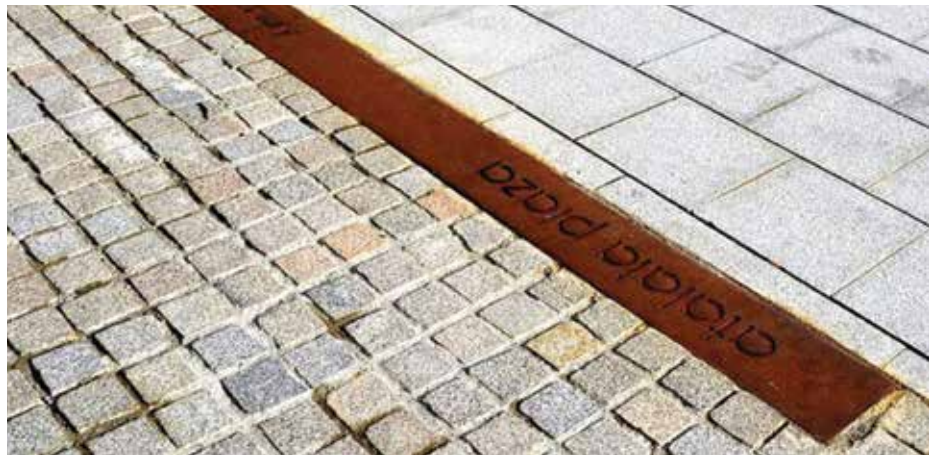
Paving and Corten marker, Arminza, Spain
